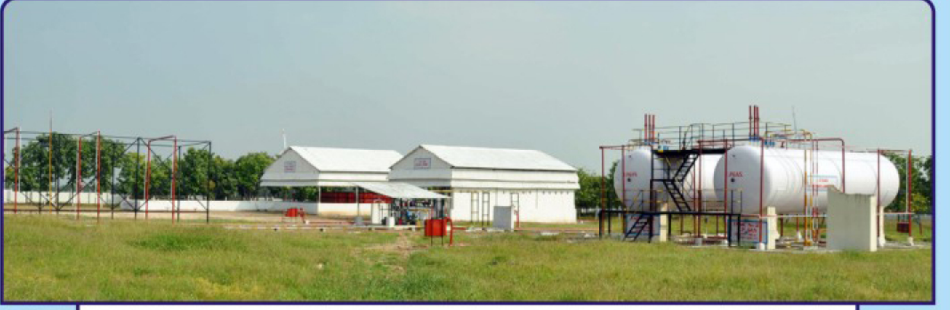
GLOA RAJAM GAS LPG BOTTLING PLANT AT KUNDADAM, TIRUPUR DIST, TAMILNADU
